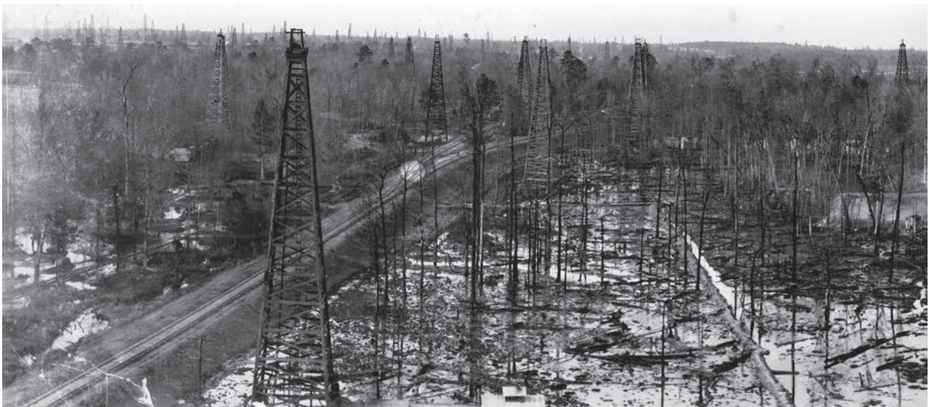
More than 75 derricks are shown drilling the field in Smackover, Arkansas, 1925. The large number of wells drilled too closely together caused damage to the natural resources above and below the surface. Arkansas Museum of Natural Resources (1985.016.001).
